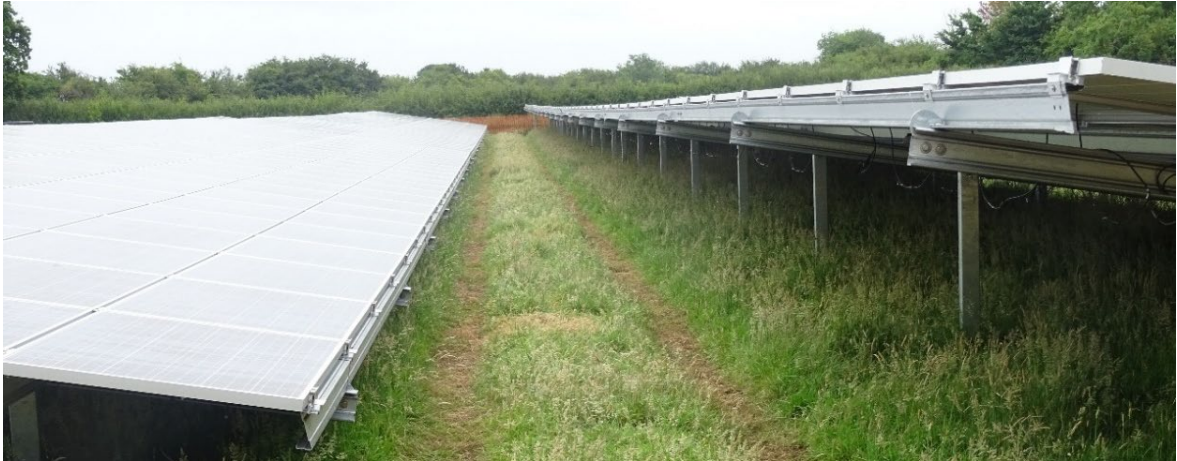
Figure 15.12 Part Installed Panels (Bentham Farm, Purton)
