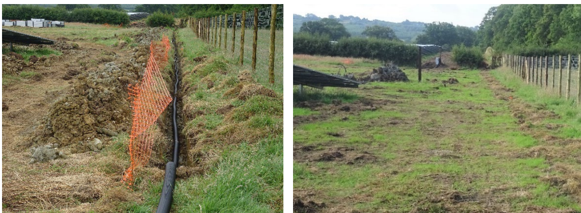
Figure 15.15 Cabling Channels during Cable Installation
