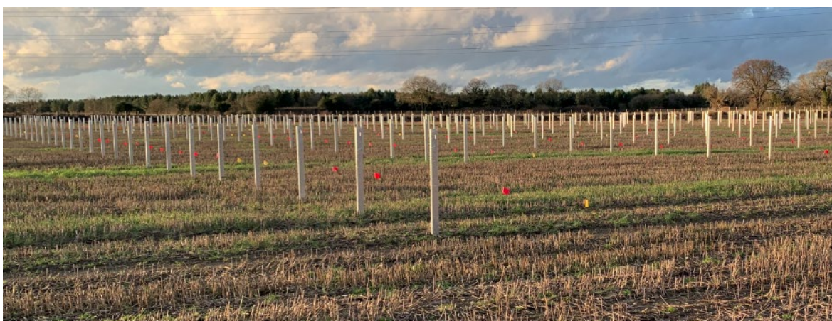
Figure 15.11 Mounting Structure Piles being Installed (taken at Tilm Farm, Retford, in January 2023)
