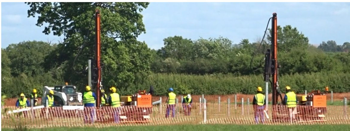
Figure 15.10 Mounting Structure Piles being Installed
